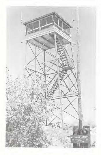
Figure 227. Mount Union lookout, an Aermotor MC-24, built in 1933 on Prescott National Forest.
